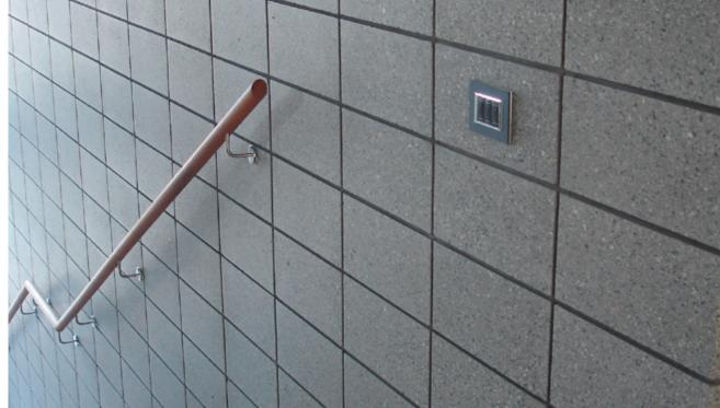
S-Protect water repellent products are used to treat dense concrete such as precast or veneer masonry brick providing a water repellant barrier to liquid water while maintaining the concrete's natural vapour permeability. The S-Protect Silane molecules are particularly small in comparison to other treatments and with a low viscosity but high concentration of active ingredients penetrate deeply into the concrete substrate rendering it hydrophobic.
